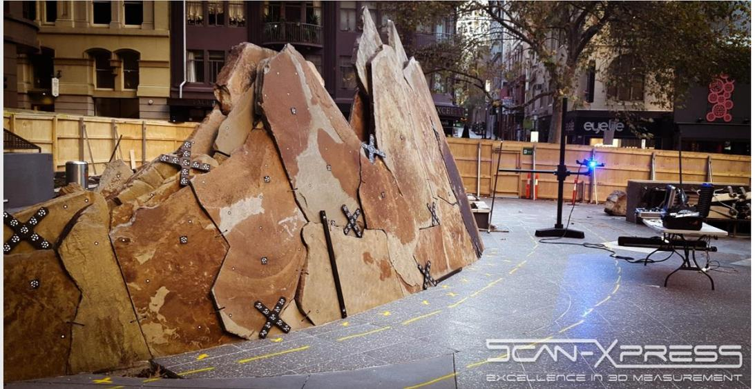
Following the photogrammetry a series of scans were taken to capture the entire outer surface of the sculpture. A model was generated which precisely located each sandstone slab. With the position and orientation of each individual piece documented the sculpture could be dismantled with confidence.
