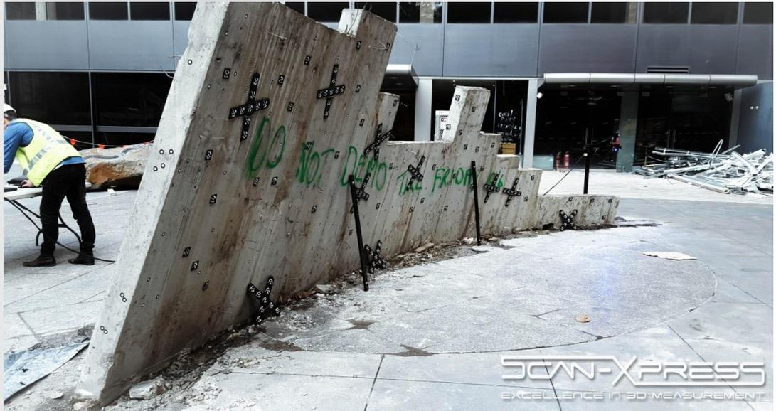
With a full scan of the concrete substrate completed it could then be demolished. Using the captured geometry an identical support structure could be fabricated at the sculpture's new location.
